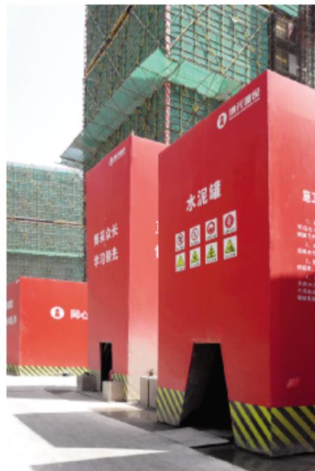
干混砂浆桶和搅拌机搭设封闭式防护棚
